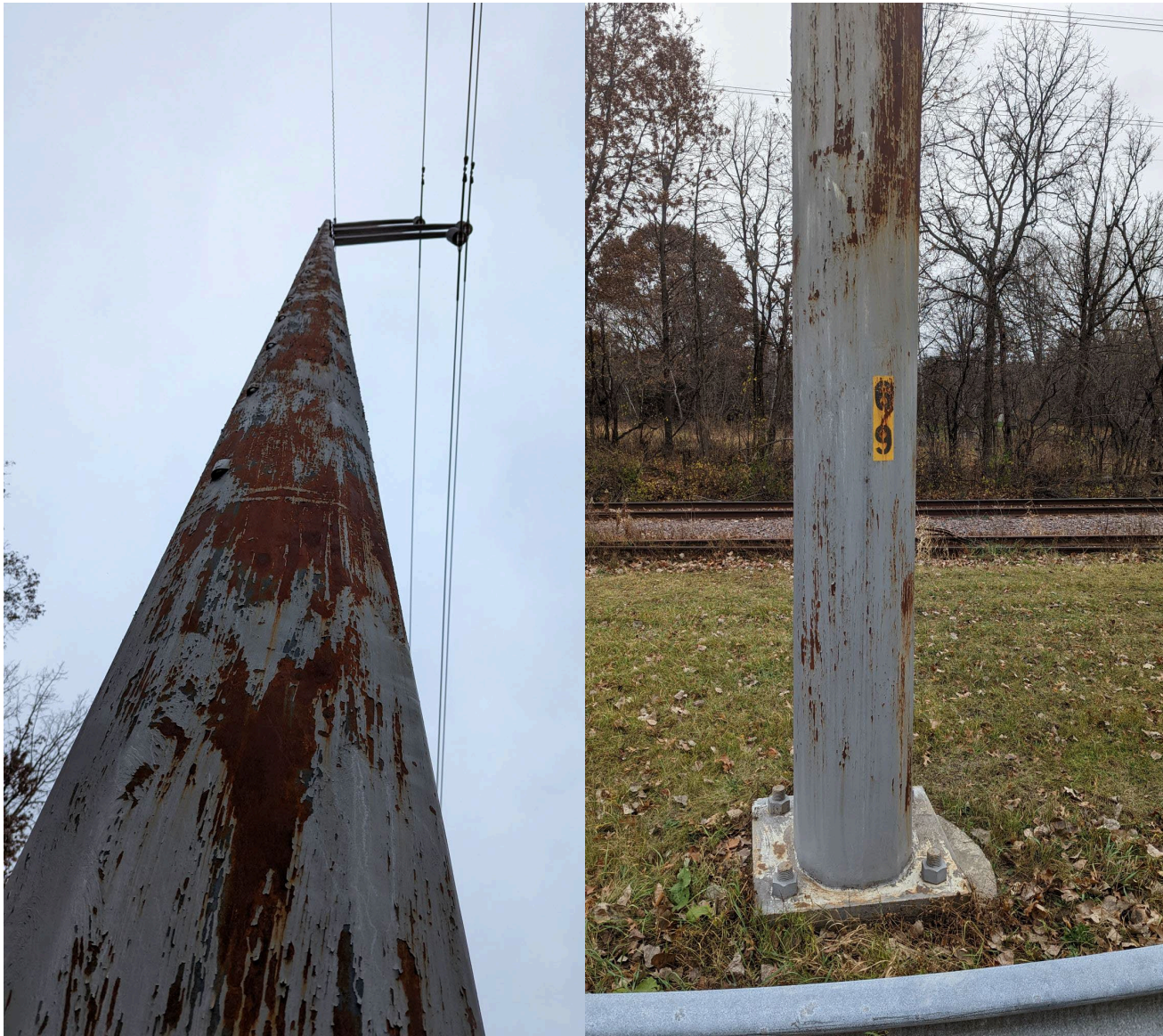
Existing Painted Poles
