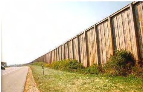
the barrier. The barrier must be high enough and long enough to block the view (line of sight) of the highway. This is the phenomenon that allows a noise barrier to provide a perceivable noise reduction. Noise barriers do very little good for homes on a hillside overlooking a road or for buildings which rise above a barrier. Openings or gaps in barriers for driveway connections or street intersections reduce barrier effectiveness.
