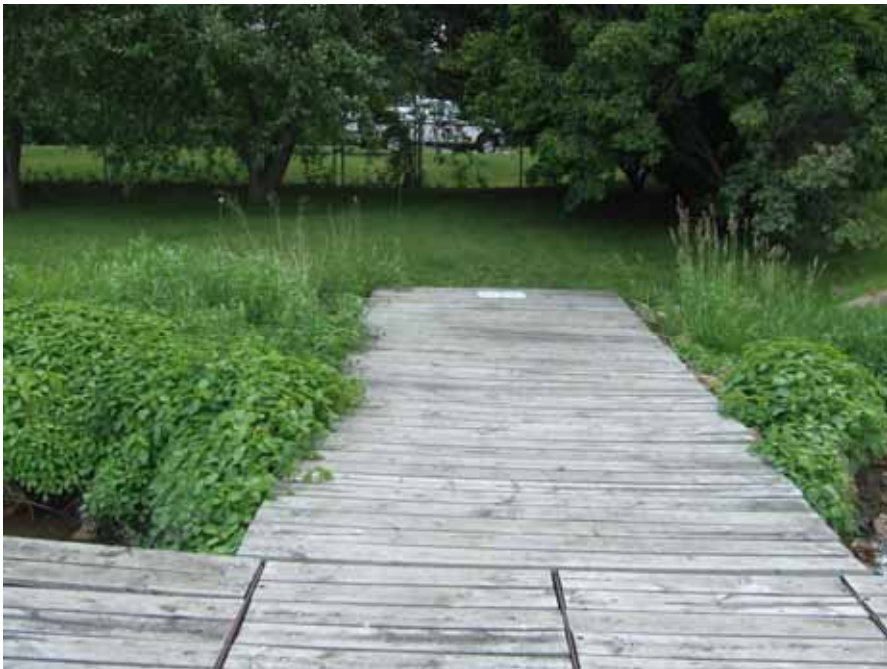
ID53: 6-6-7 003 – As-built 441 toward Owasso Blvd. N
