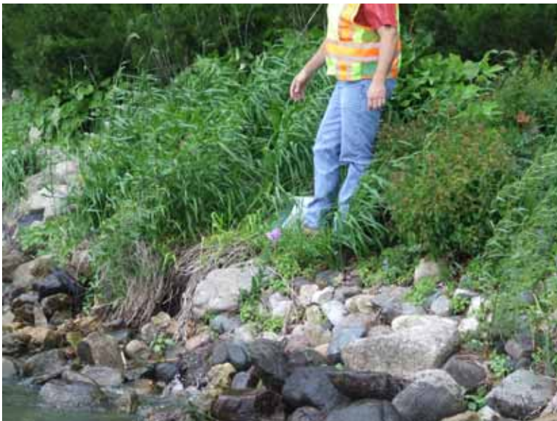
ID39: 3328/3320 Owasso Heights Road – 12” PVC (City owned. Will be converted to just an overflow during reconstruction of the road this summer. A 100,000 gallon storage tank, stormceptor and lift station will be installed to handle 80-90% of the storms, only the really heavy storms water will drain to the lake, but after the stoorage tank is filled.)
