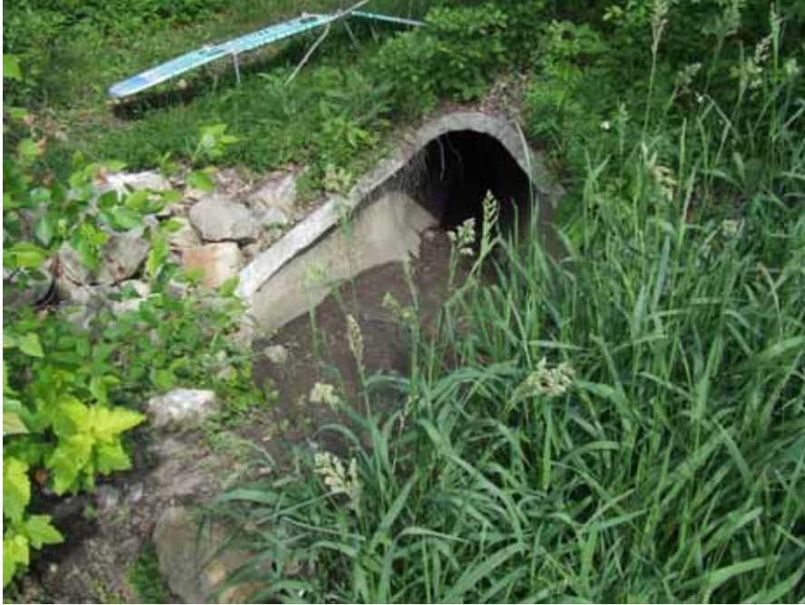
ID38: 6-6-7 001 – Outlet for as-built 372. Owasso Blvd. N near Kent Street
