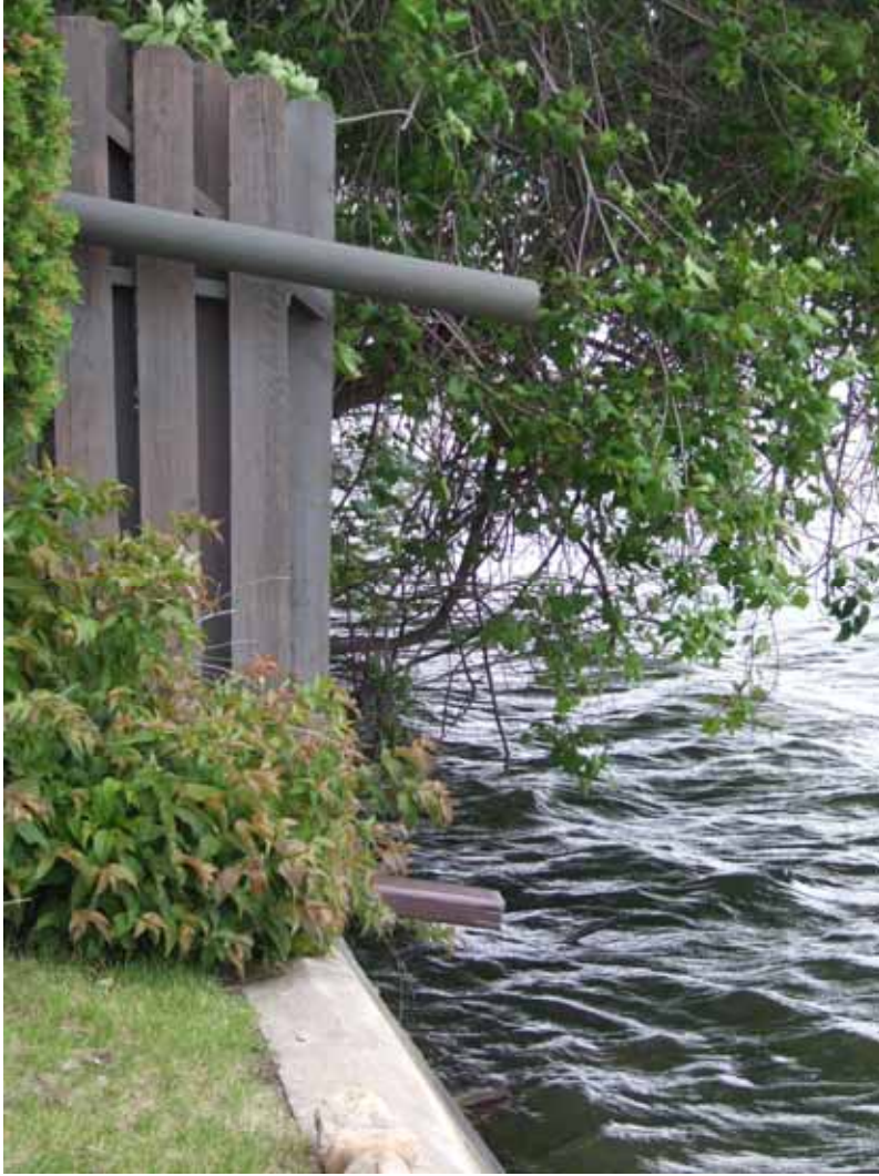
ID46: 3240 Owasso Heights Road – 6” PVC and roof drain downspout
