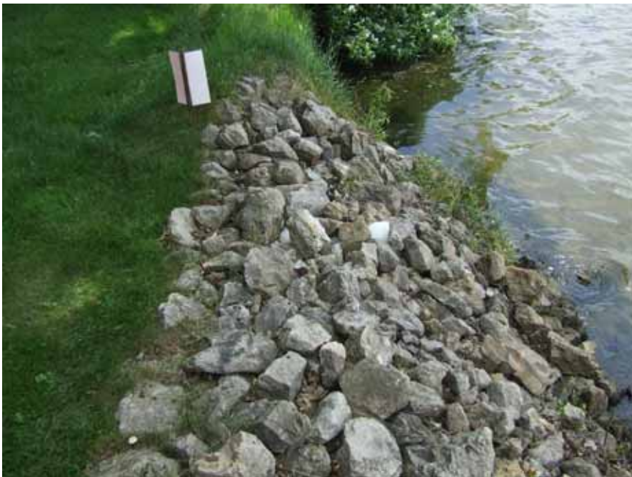
ID36: 6-4-7 011 – Outlet at 206 Woodbridge Street
