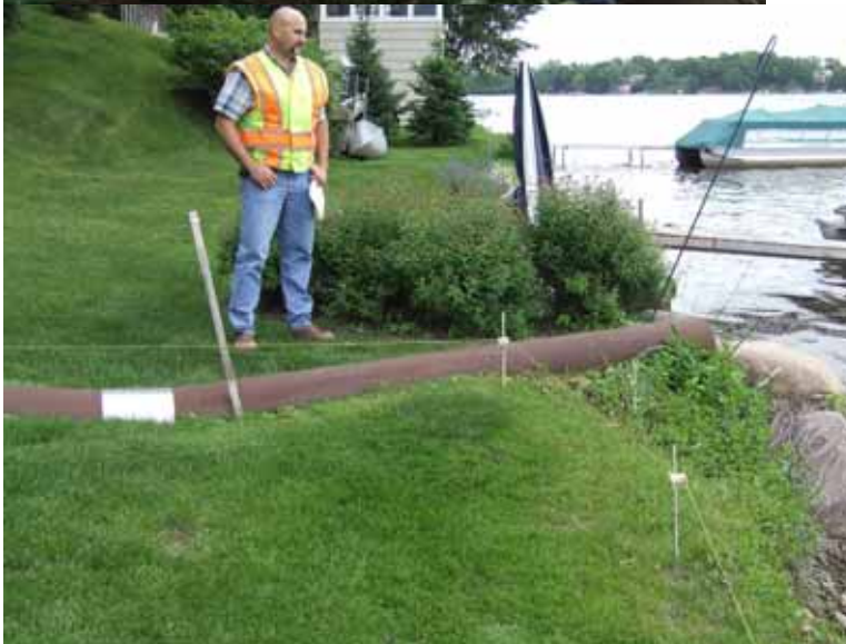
ID50: 3194 West Owasso Blvd. – 12” steel pipe (installed by either Ramsey County or the City many, many years ago. The pipe was capped at the road during a reconstruction project, so no water from the street drains through it. There are, however, a couple inlets and holes in the pipe that the water from the yard and driveways drain in to.)
