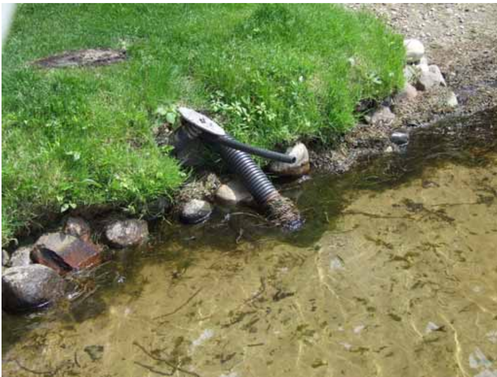
ID41: 212 East Owasso Lane – 2 – 6” flexible plastic
