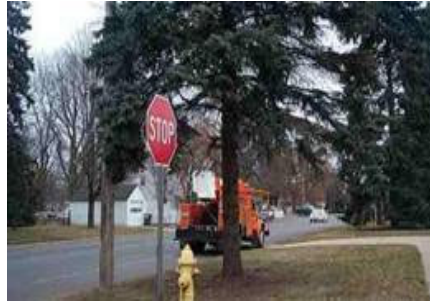
Improved visibility at traffic control sign
