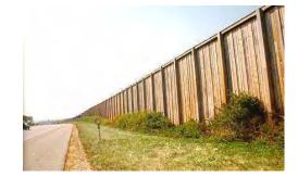
the barrier. The barrier must be high enough and long enough to block the view (line of sight) of the highway. This is the phenomenon that allows a noise barrier to provide a perceivable noise reduction. Noise barriers do very little good for homes on a hillside overlooking a road or for buildings which rise above a barrier. Openings or gaps in barriers for driveway connections or street intersections reduce barrier effectiveness.
