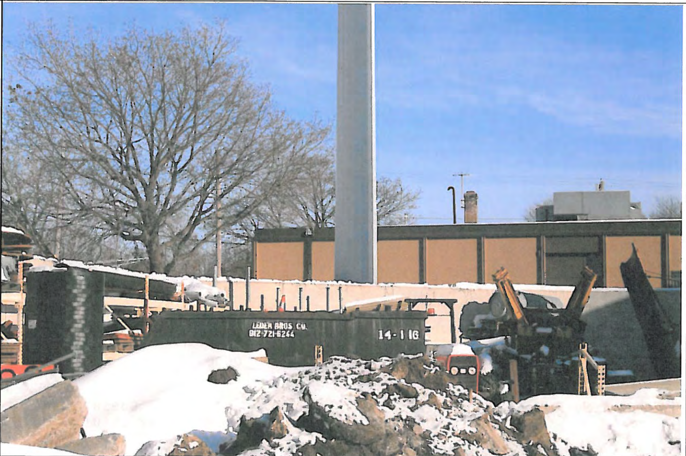
SITE 2 - Civic Center Campus Pole – Base section of 150' pole at ground view in yard.
