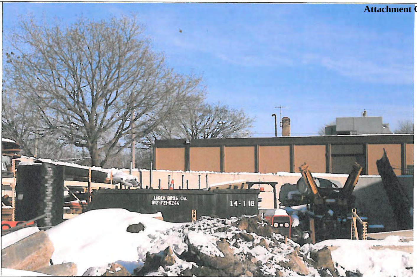
SITE 2 - Civic Center Campus Pole – Current View from Public Works Yard
