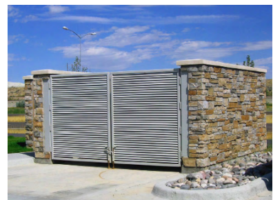
Trash-storage enclosure with masonry walls
