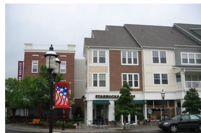
Window and door openings.
