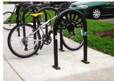
The City encourages the use of the "inverted U" type bike rack. Bike rack designs should provide for:
