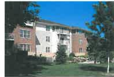
Building with street-facing facade articulated by offsets, changes in materials, and window placement
