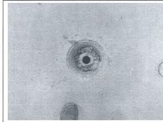
Facing: Down View of: Dry floor drain in basement
